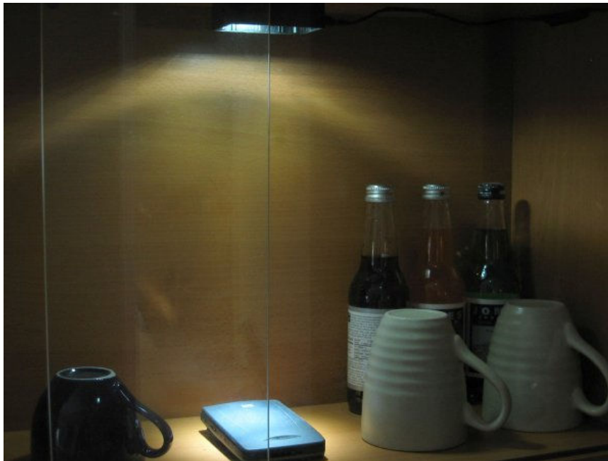
The LLIA90 LED illuminator mounted inside a cabinet for décor lighting. The power supply can be connected to a power switch for manual on/off operation.
